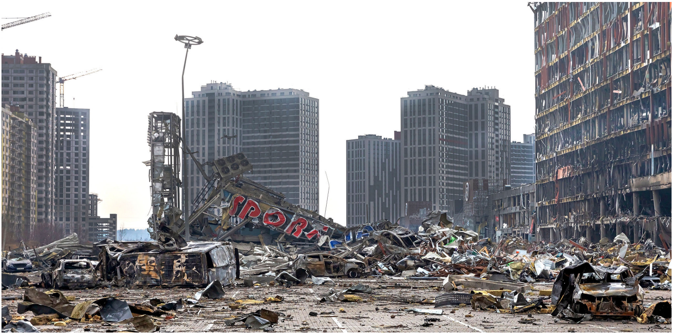
Damaged shopping center in Kyiv. Credit: Adobe Stock
